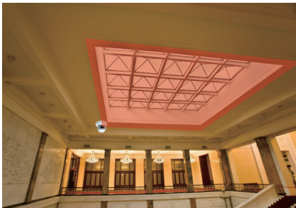
Skylight protection at Public facility / Warehouse
